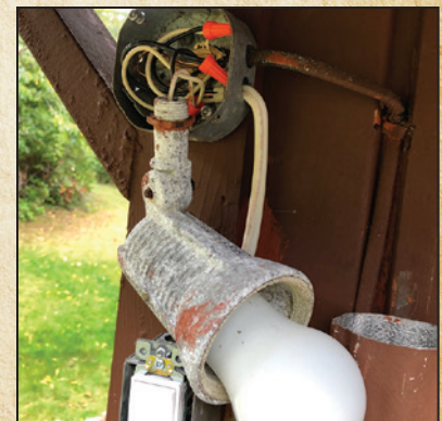
Exhibit A: Exposed wires and substandard workmanship
